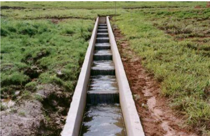
Figure 3. Concrete spillway channels to allow excess water flow between ponds.
